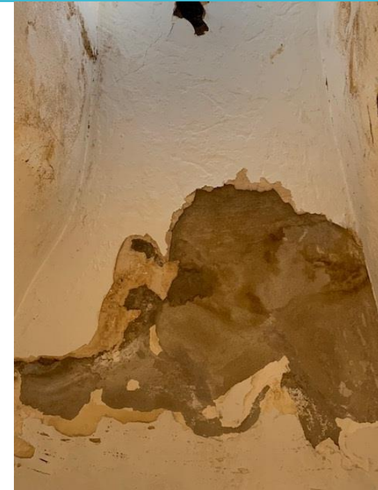
Ceiling, Town Hall
